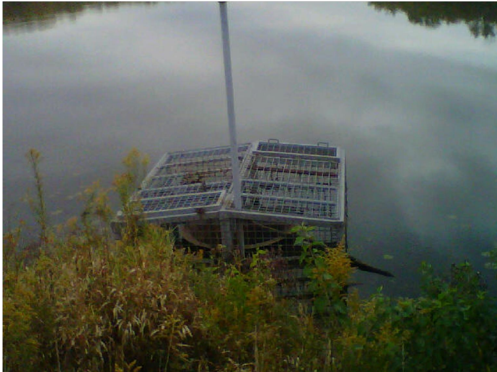
Morning Glory Structure with Trash Rack
