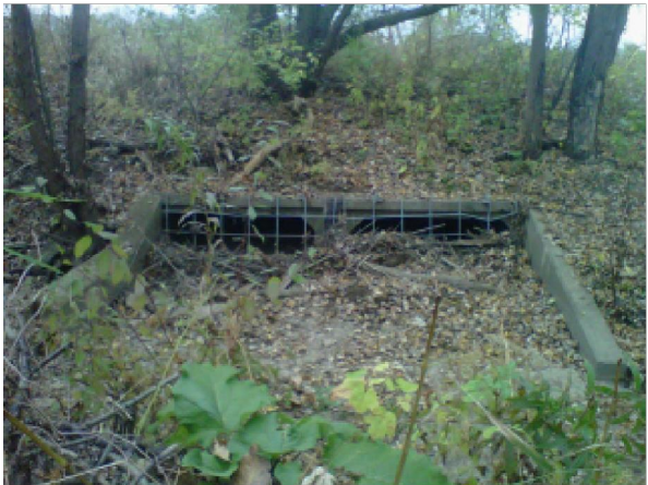
Inflow at Upstream End to Sediment Basin B
