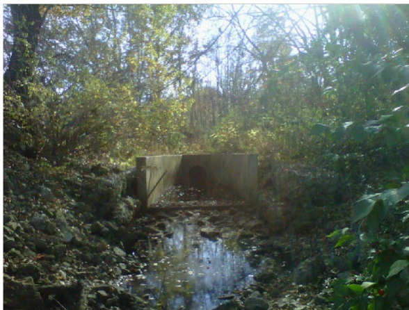
Morning Glory Structure with Trash Rack
